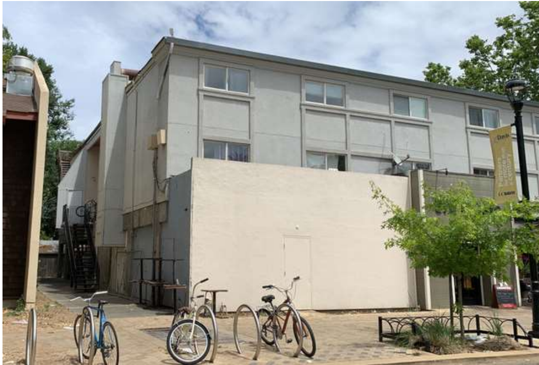
West and south facades, ESA 2022
