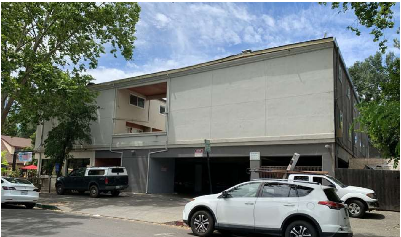
East façade, ESA 2022
